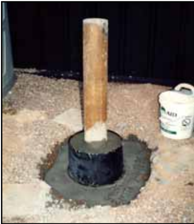
Pier was put in on July 1, 1996
