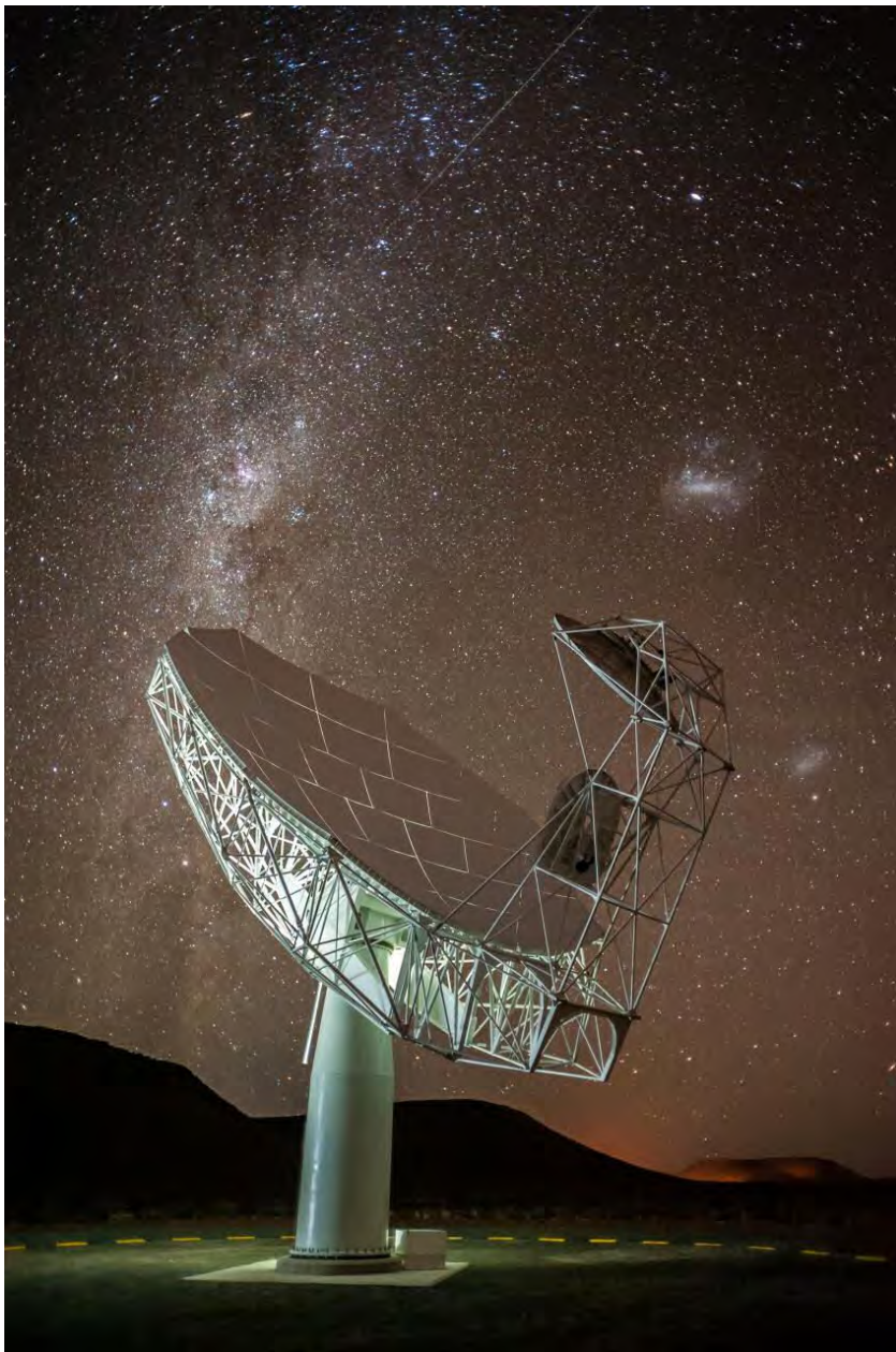
Figure 4: MeerKAT One of the 44.3-foot-diameter MeerKAT radio telescope dishes located in the semi-desert Karoo region of South Africa. The off-axis parabolic dish focuses the radio waves toward the off-axis secondary, which sends it on to the waveguide front-end of the receiver. The full MeerKAT array will consist of 64 identical antennas. The MeerKAT array is a precursor to the Square Kilometer Array (SKA).
