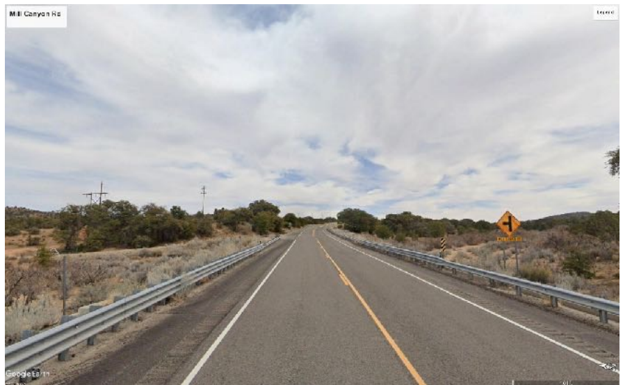
Route 90 at Mill Canyon Road
